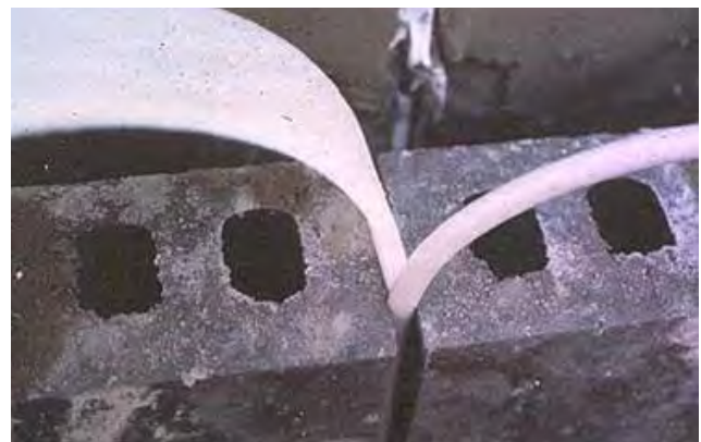
Photo 1 Vertical Expansion Joint Construction
